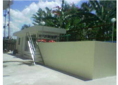
Pharmaceutical Laboratory SBR Process Capacity: 48 m 3 /day
