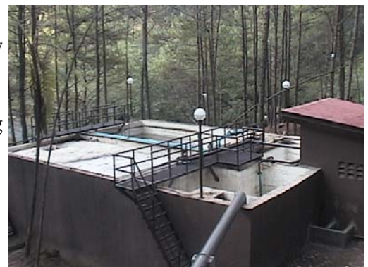
Commercial, Convention and Entertainment Center SBR Process Capacity :300 m 3 /day.
